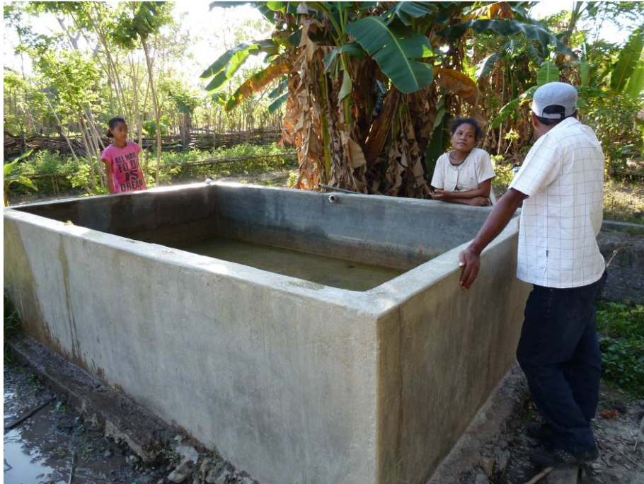
Figure 2: A concrete water tank built by a group in suco Maubaralissa
