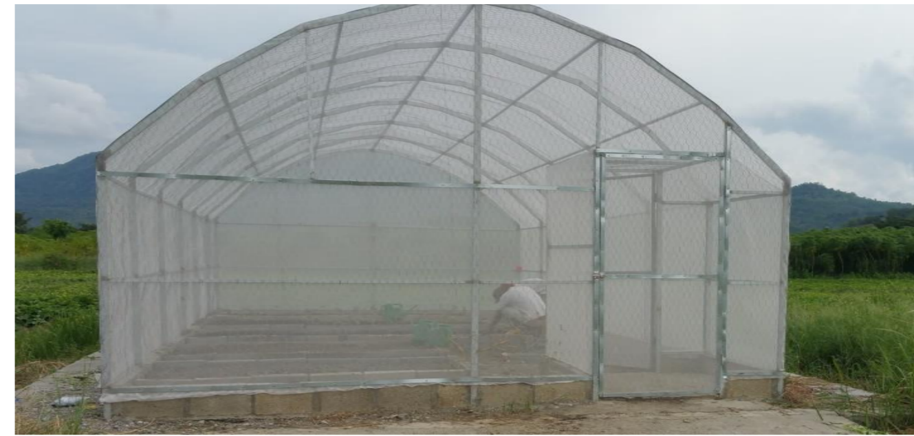
Figure 1. Screen house to prevent virus vector and other insects at Loes research Station
